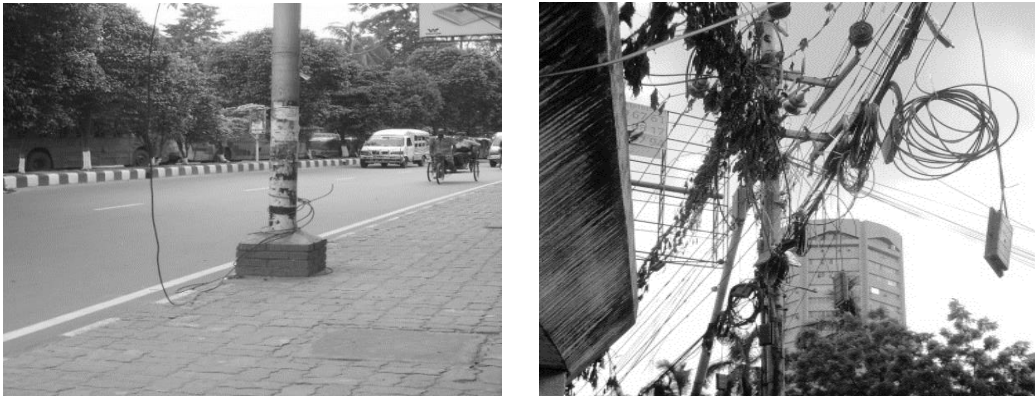
Figure 4: Electric wire on the pavement (source: Barua et al., 2007)
